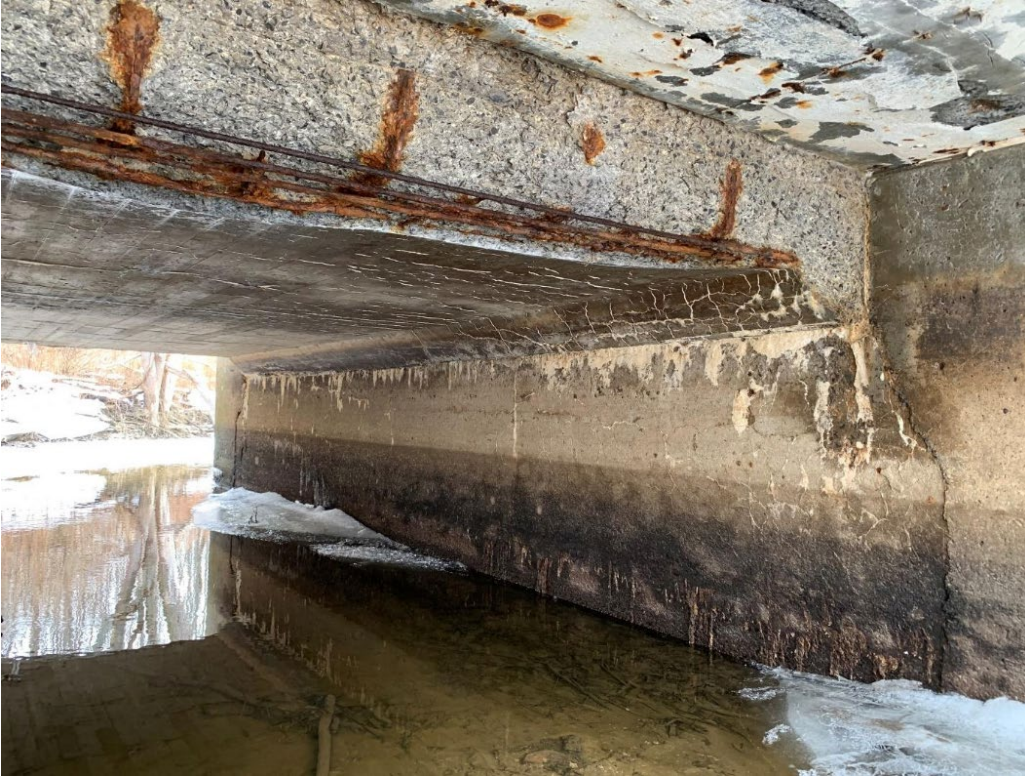
Looking upstream from inside structure at outlet
