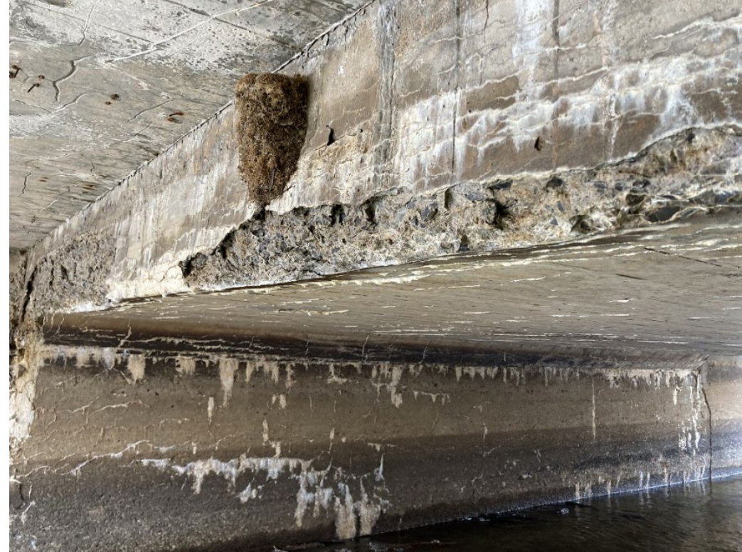
Inside structure at inlet
